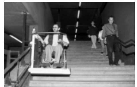
In accordance with the space and financial resources available, access to the stations is possible through a lift (Barcelona) or a stairlift (Milan)
